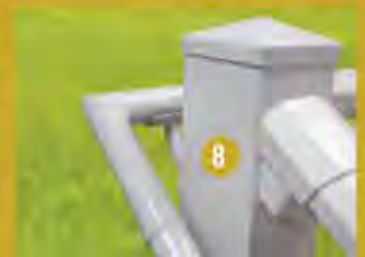
90° Welded Elbow Detail
