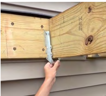
Double-Shear Nailing
